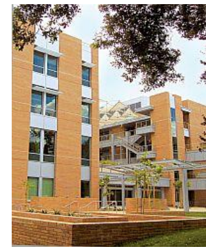
UCR Engineering Building
